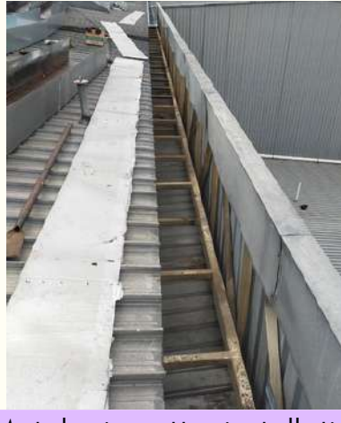
Metal rain gutter installation
