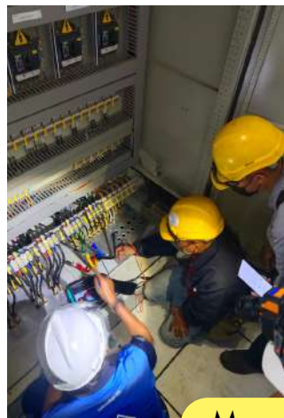
Incoming cable installation
