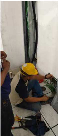
Megger insulation test
